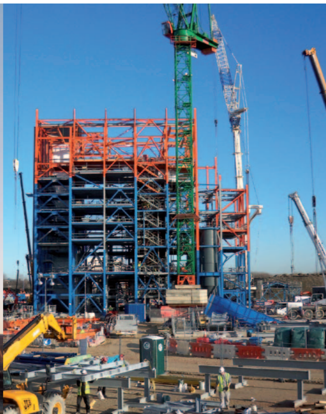
Stair tower and boiler building
