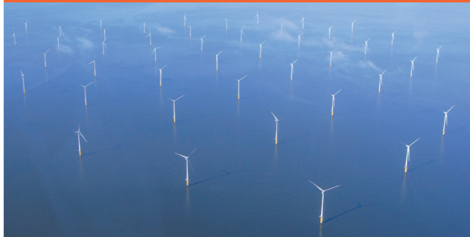
Robin Rigg Offshore Wind Farm
