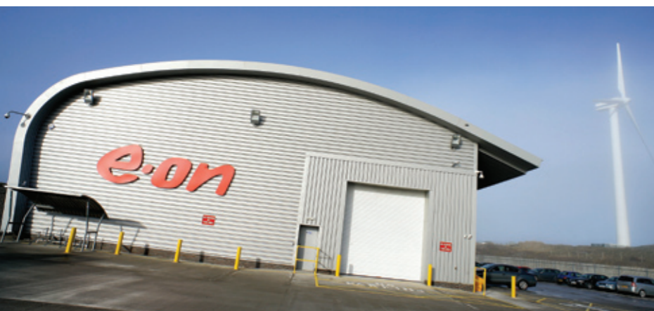
Robin Rigg Operations and Maintenance building, Port of Worthington
