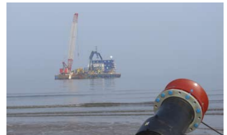
Above: The barge in action laying the cables
